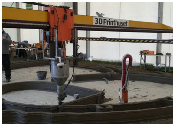
Fig. 2 Contour crafting printing using a gantry-based system [11]
