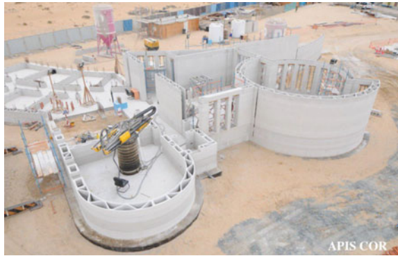
Fig. 8 Construction of 3D printed office in Dubai [40]
