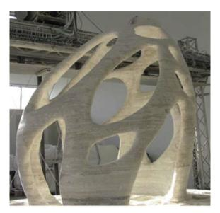
**Fig. 3** Structure printed using the D-shape method [4]
