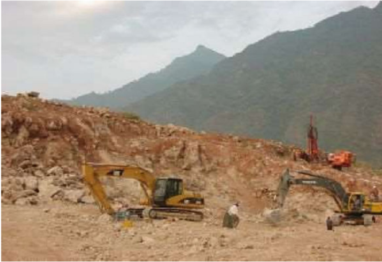
Fig. 2 Actual strata at Spillway during excavation
