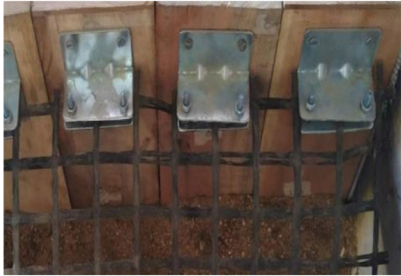
Fig. 5 Mechanical connection between facing panel and geogrid
