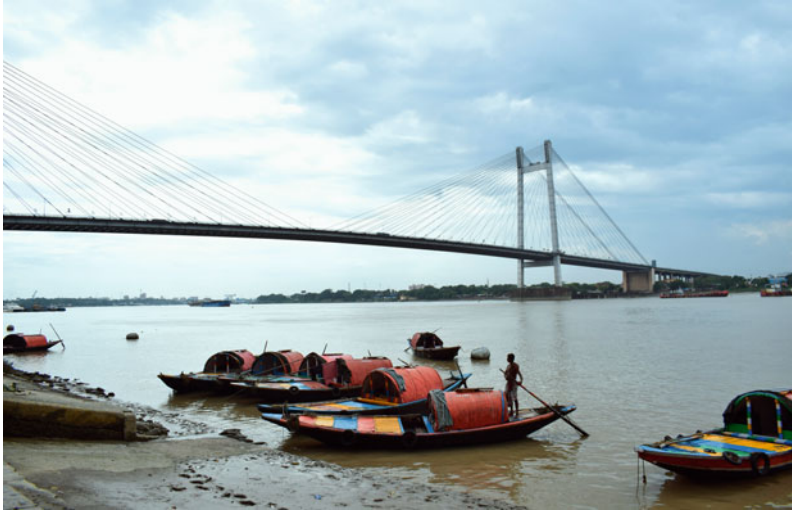
Fig. 14 Vidyasagar Setu or the Second Hooghly Bridge, completed in 1992, is situated at south Howrah Bridge and is considered to be a piece of modern design with the bridge hanging on ropes from the four towering pillars standing on both sides of the river. Picture credit: Amir Khan
