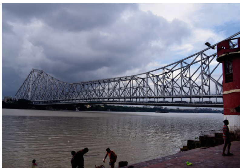
Fig. 13 Connecting Howrah railway station in the west and Barabazar in the east across the river Hooghly, Howrah Bridge or the New Howrah Bridge or now called Rabindra Setu completed in the year 1941 is a marvel of engineering expertise and happened to be the main gateway to Kolkata. Its magnificent hanging cantilever structure made of steel plates and bolts is a wonder in itself, and it is a testimony to the identity of the city of Kolkata. Picture credit: Asrafal Alam
