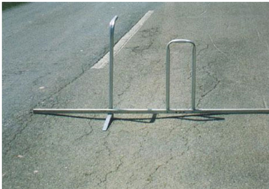
Fig. 3 Manual measurement of rutting using a straight edge
