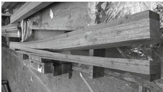
Fig. 7 Glulam beam sample A (Control) after failure at maximum load
