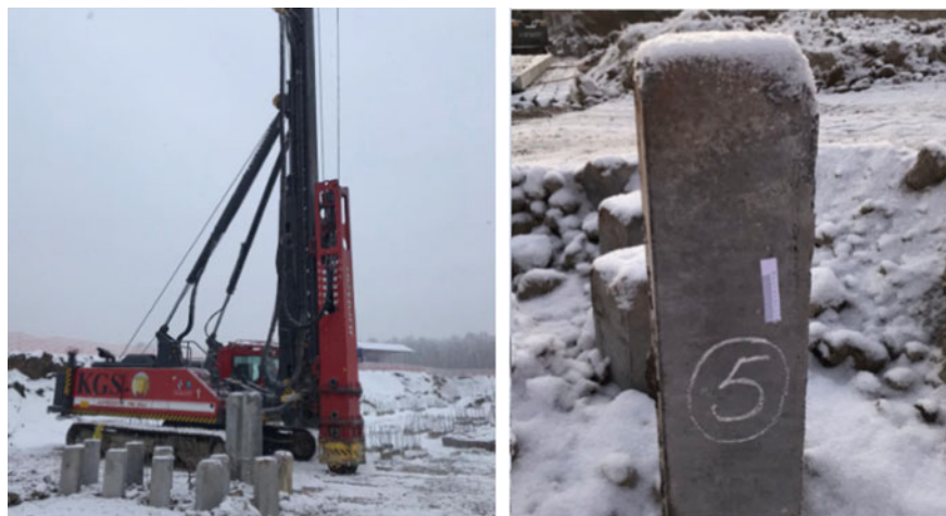
Fig. 2 a Junttan PM-25HD piling rig. b Typical test pile
