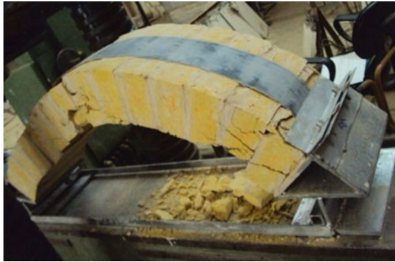
Fig. 20 Strengthened arch, material spalling
