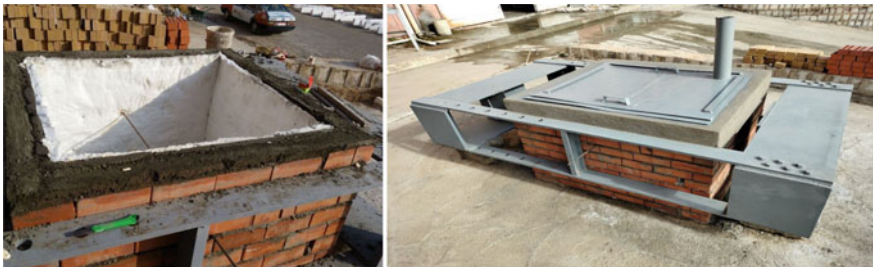
Fig. 9 Steel frame and incineration oven
