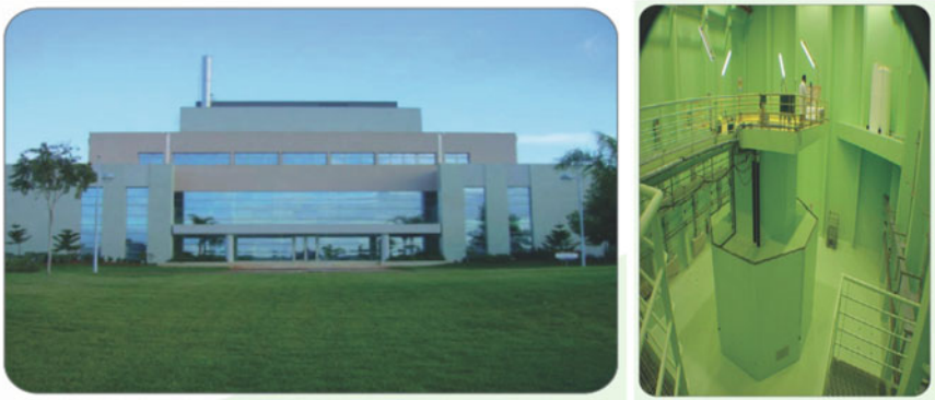
Fig. 4.23 MA-R1, 2 MW building and reactor hall, Morocco [10, 27]
