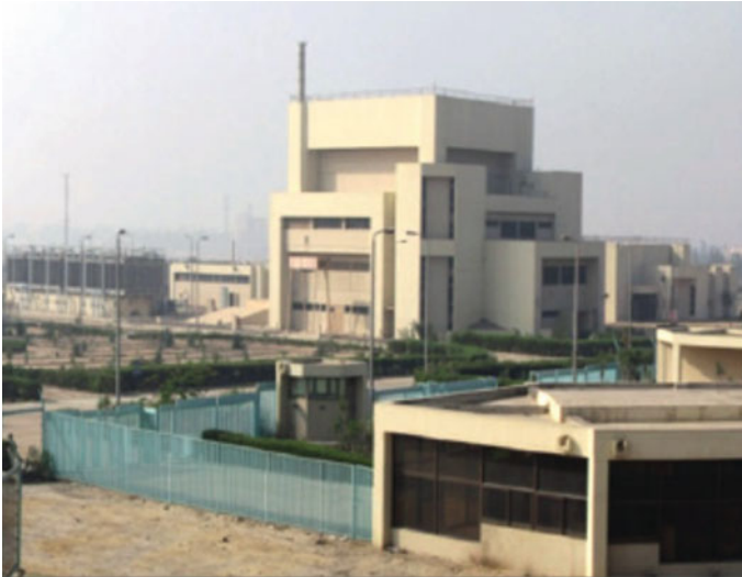
Fig. 4.13 ETRR-2 reactor facility, Egypt [27]
