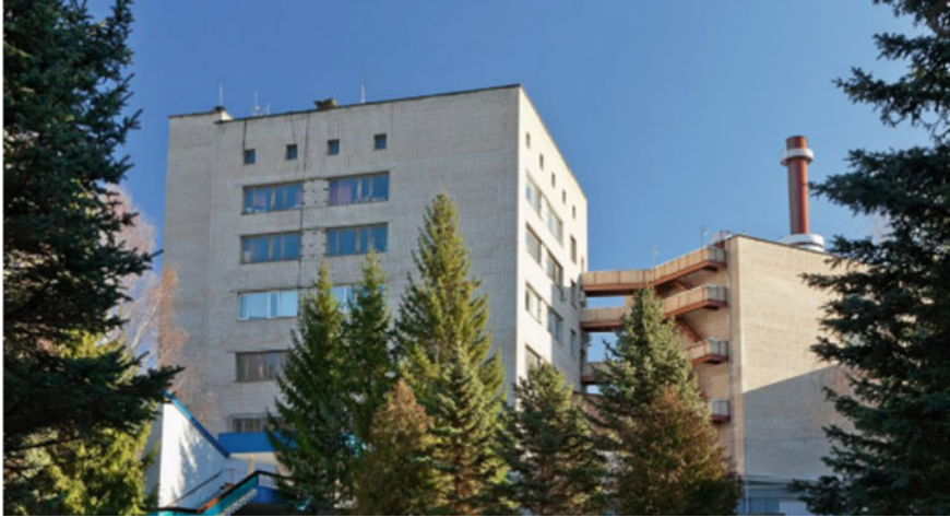
Fig. 4.27 IBR-2 reactor building, Russia [57]
