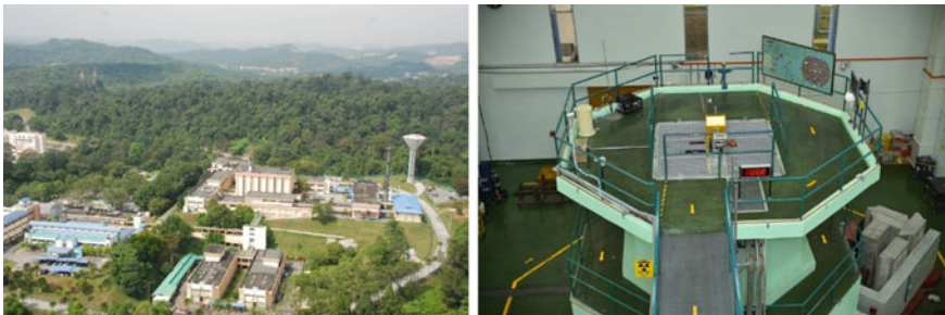
Fig. 4.22 TRIGA II PUSPATI 1 MW facility and reactor hall with neutron imaging beamline, Malaysia [47]
