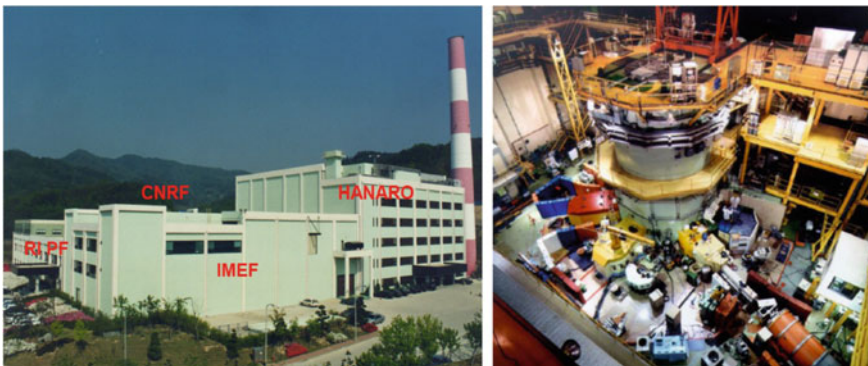
Fig. 4.21 HANARO reactor building and hall, South Korea [46]
