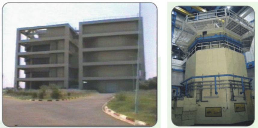
Fig. 4.5 Nur facility and reactor block, Algeria, Africa [27]
