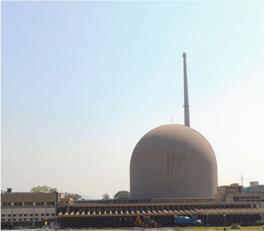
Fig. 4.45 CIRUS reactor facility
