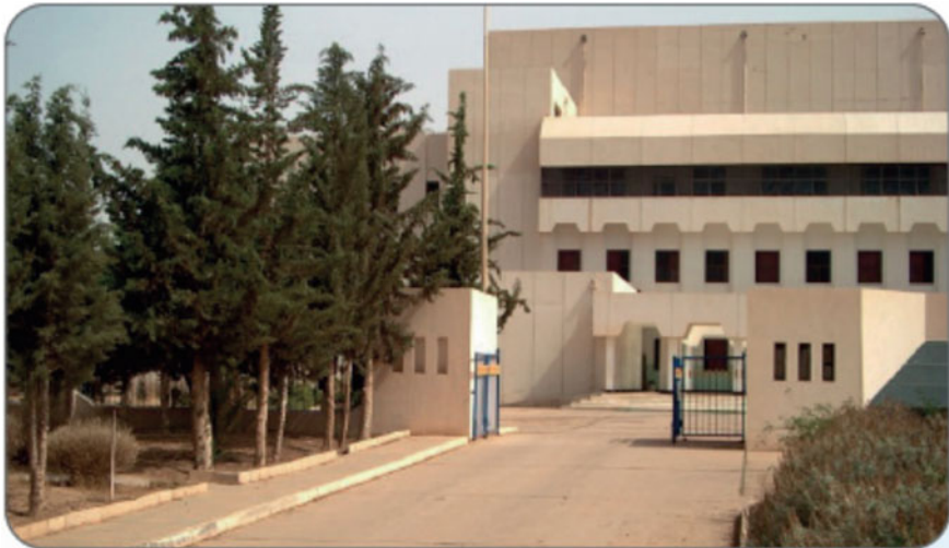
Fig. 4.4 Es-SALAM reactor building, Algeria, Africa [27]
