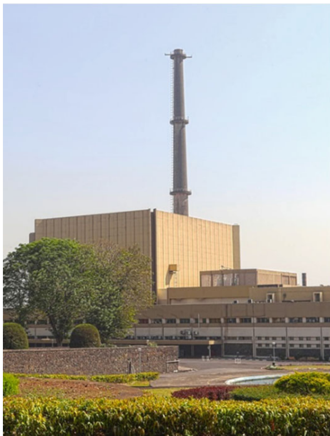
Fig. 4.47 Dhruva reactor facility
