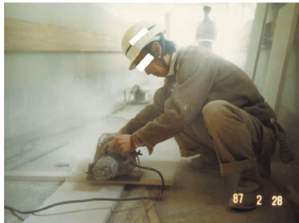
Fig. 9.1 Heavy dust exposure to a carpenter during cutting asbestos-containing board with an electric circular saw at a construction site in 1987. The airborne asbestos (type: amosite) concentration of 131 \times 10^3 f/L at his respiratory zone, corresponds to 873 folds of the current administrative level (150 f/L) of asbestos in Japan
