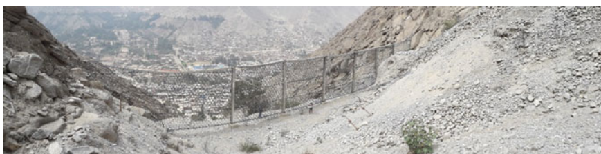
Fig. 3 Flexible barrier of the Carossio creek
