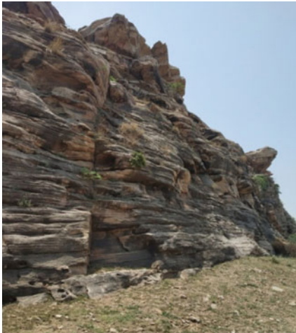
(a).North – West slope, indicate High Hazard, Toppling failure
