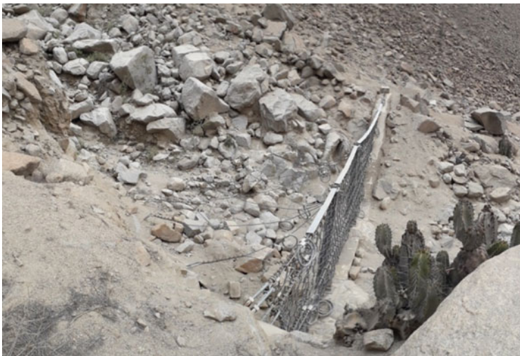
Fig. 7 Volume of solids retained in the Castilla debris flow barrier in 2017
