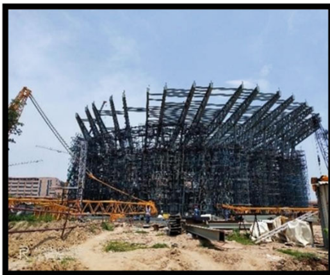
Fig. 2 Front View of Convention Centre
