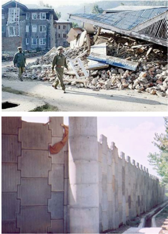
Fig. 3 (Top) Damage sustained by buildings in Uri 30 km from site and (Bottom) MSE approach wall for Bridge No. 127 after the earthquake [5]
