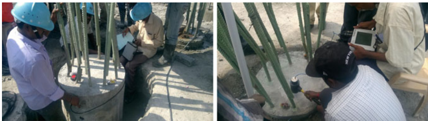
Fig. 1 UPV testing and pile integrity testing on a typical pile
