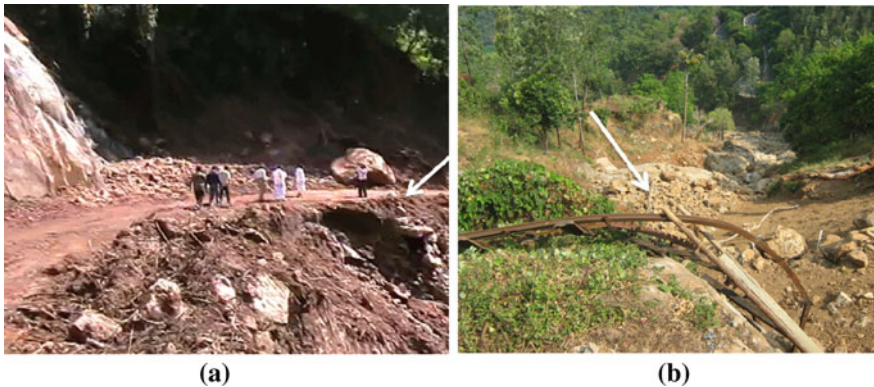
Fig. 4 View of Marappalam 2009 landslide. a View of damaged road network b Damaged railway track and debris materials along the run-out distance [13]
