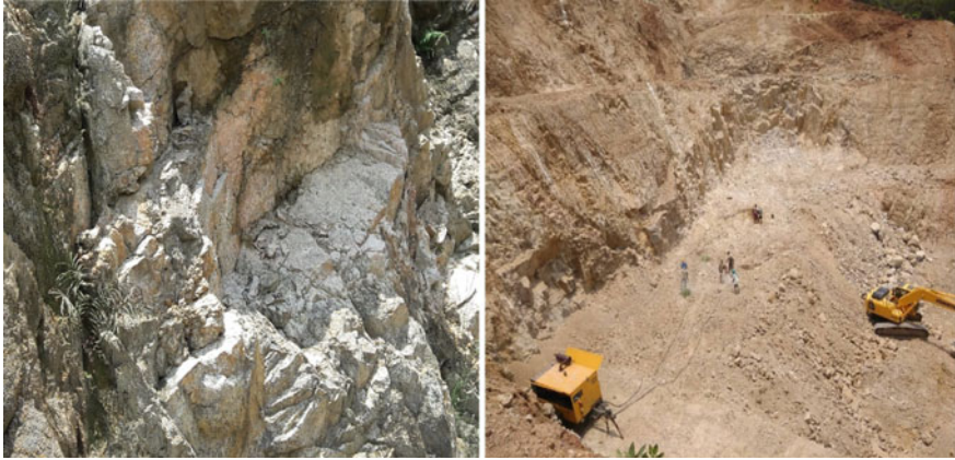
Fig. 2 Site Photos at approach of left irrigation tunnel of Polavaram
