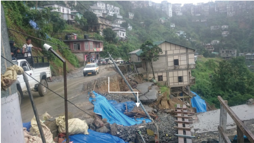
Fig. 4 Sinking/sliding of national highway
