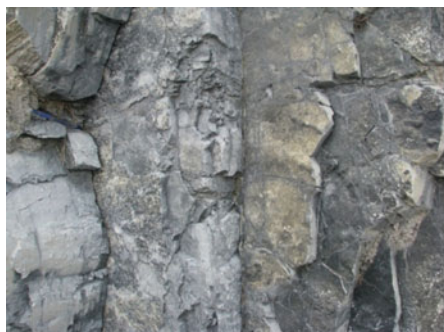
C) Rough and smooth undulated bedding joint surfaces
