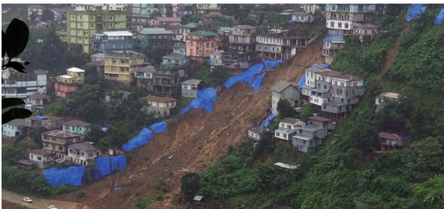
Fig. 3 Affected area above national highway
