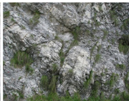
G) Joint apertures having soft infilling material with grown grasses
