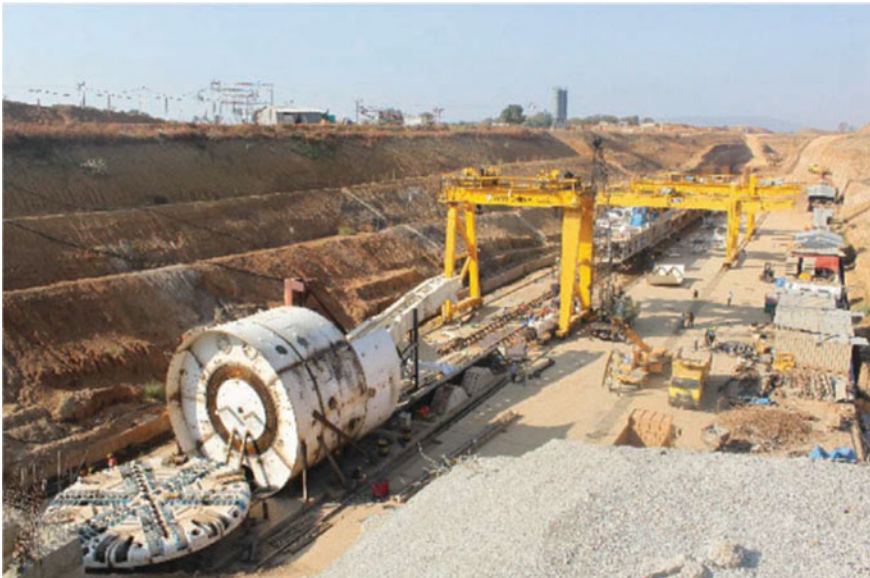
Fig. 2 Onsite assembly of TBM
