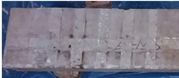
Fig. 2 Surface preparation for JP0
