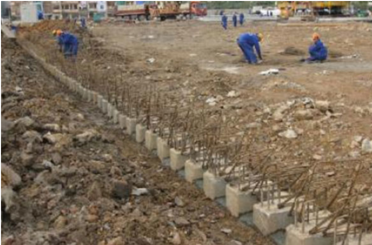
Fig. 6 Construct the top-wall girder
