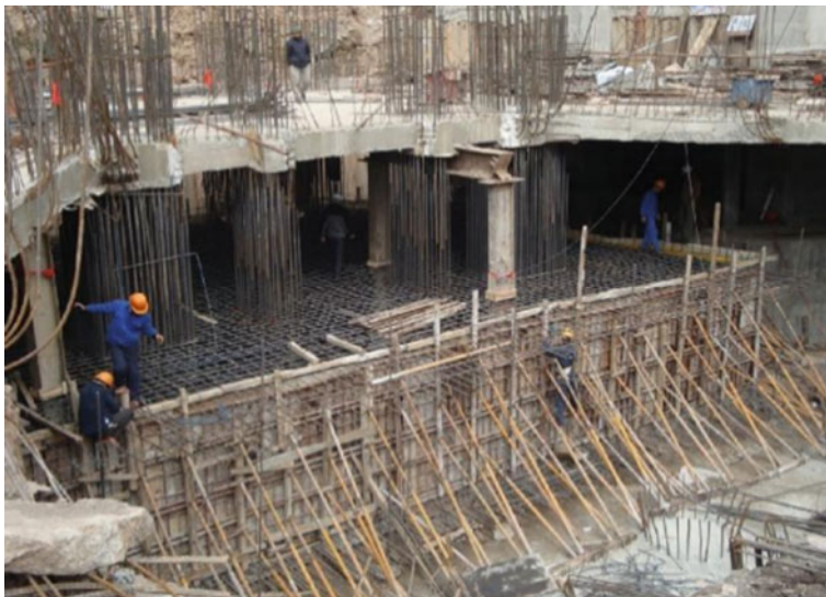
Fig. 10 Construction of foundations, foundation beams
