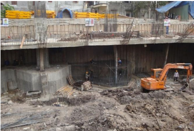
Fig. 9 Dig soil to the bottom of the foundation height
