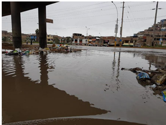
Fig. 2 Mateo Pumacahua Av. was flooded by heavy rains that fall in the districts of Villa María del Triunfo and Villa El Salvador. September 2018
