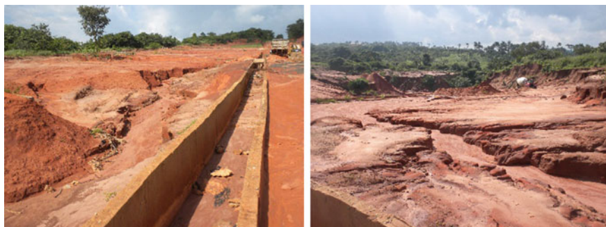
Fig. 4 Increase in gullying due to structures constructed during the reinstatement of the highway section at Km 11, Umunnekwu, Isuikwuato
