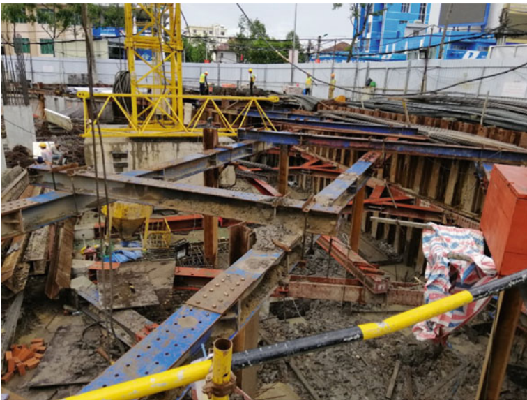
c) Open method of excavation
