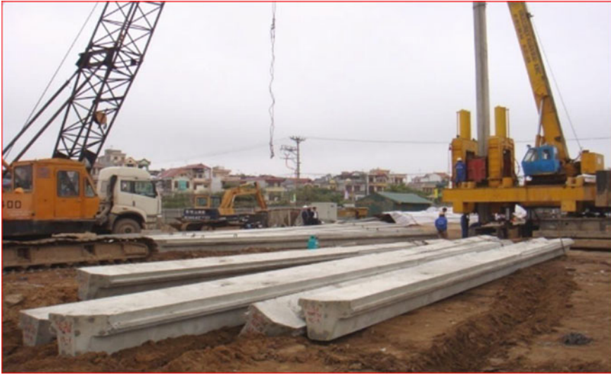
Fig. 4 Construction of pile pressing
