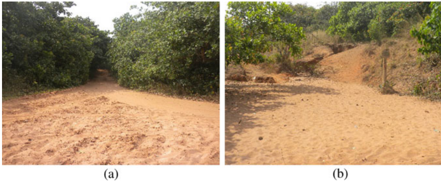
Fig. 3 a Earth road as erosion channel at Km 0.25, beside ABSU fence, Uturu. b Footpath as erosion channel at Km 13.7, NNPC Pipeline, Amiyi, Isuikwuato
