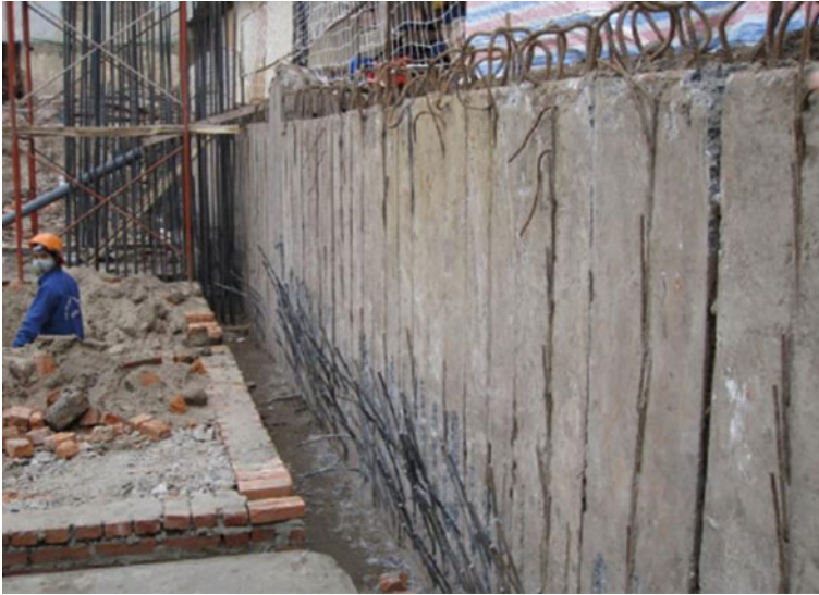
Fig. 8 Construction of beams, floors for basement 1
