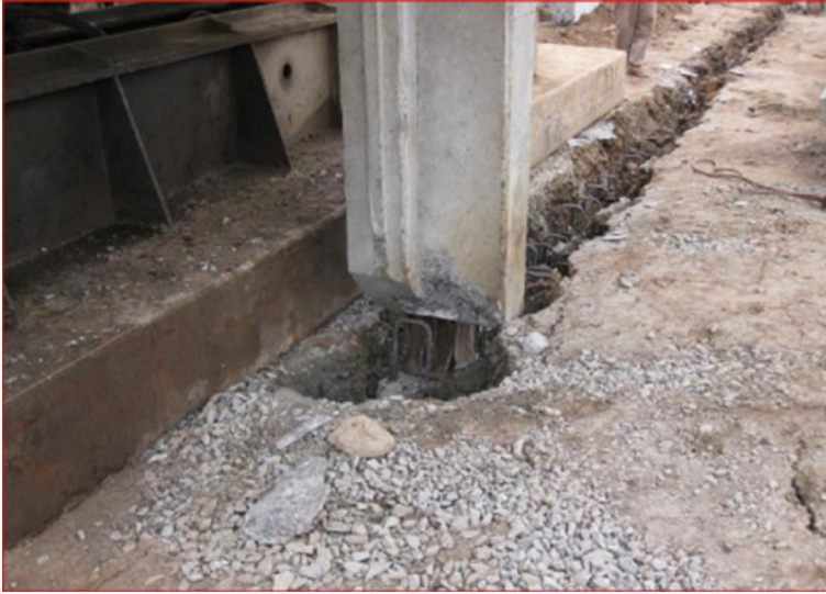
Fig. 5 Pile segments 2,3, etc., is repeated
