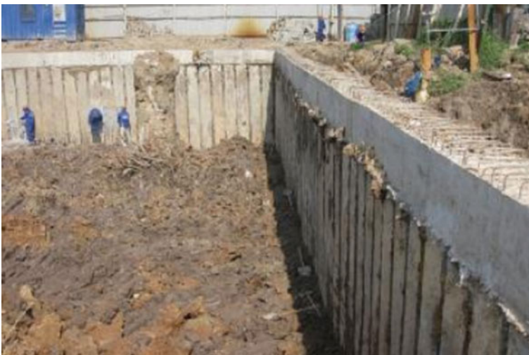
Fig. 7 Dig soil to the height of the first basement
