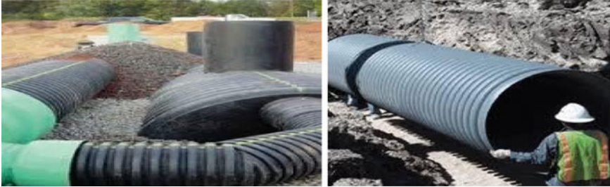
Fig. 10 Manifold piping
