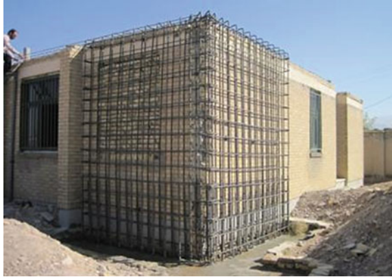
Fig. 24.6 Retrofitting URM School buildings with shear walls [10]
