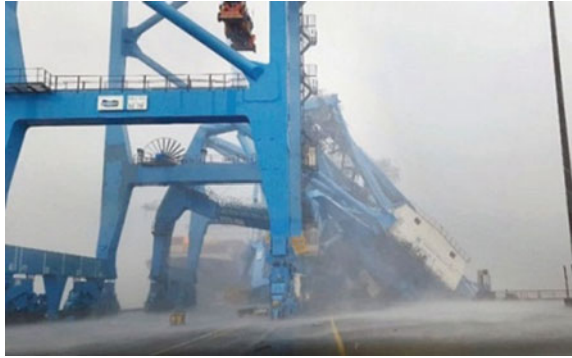
Fig. 25.4 Failure of material handling cranes in industry
