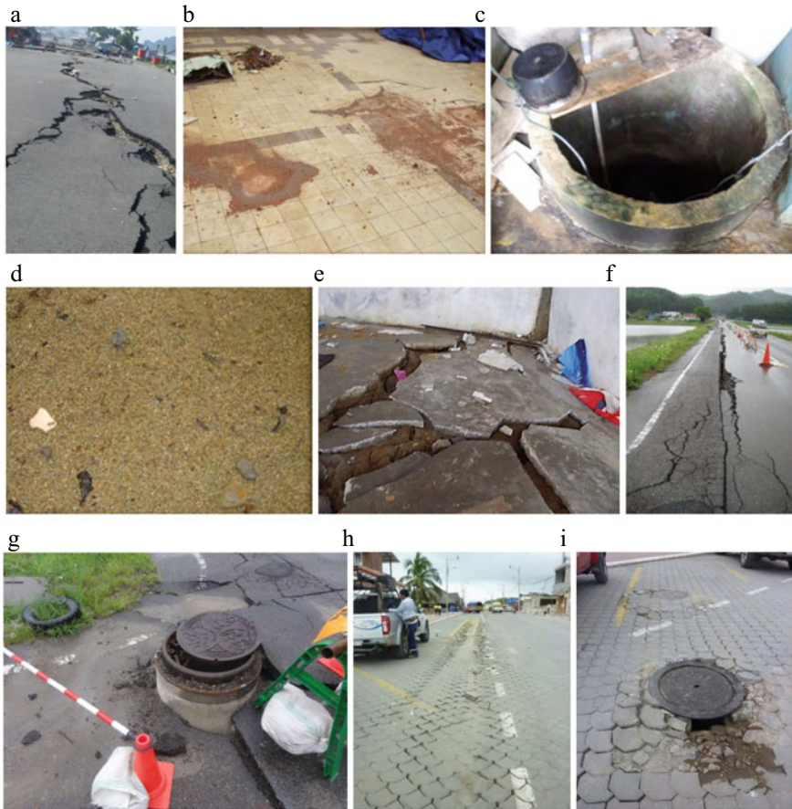
Fig. 14.10 Consequence of soil liquefaction following the Padang, Tohoku and Muisne earthquakes. a Tension cracks arising from lateral spreading at Padang city. b Sand boils in adjoining building of Mere Amelie Church, Padang. c , d The well that was blocked with sand due to liquefaction at Siteba Village, Padang. e Upheaval of floor slabs of village house due to liquefaction at Perumdram Village, Padang. f , g Uplift of manhole and lateral spreading at Shirakawa. h Ground settlement on pavement at Pedernales. i Uplift of manhole close to the observed ground settlement at Pedernales
