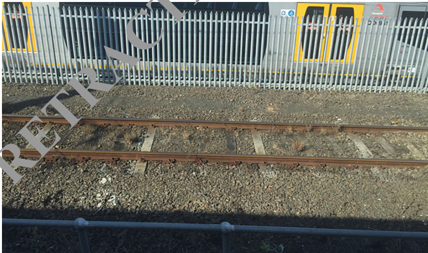
Fig. 19.2 Example of one in four interspersed tracks (one concrete sleeper after three timber sleepers—a set of four)
