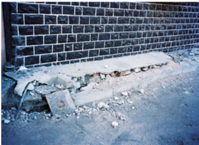
a Settlement of ground due to liquefaction. b Sand boils observed near Kandla port
