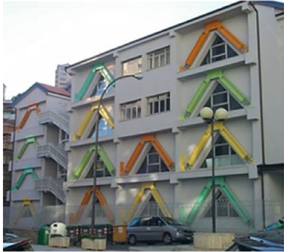
Fig. 24.10 Seismic retrofit of school buildings in Italy using ED devices shown on the outside [14]
