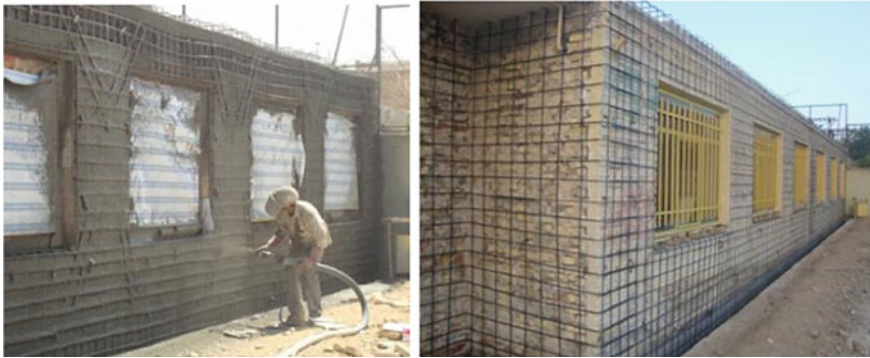
Fig. 24.7 Retrofitting single story URM school buildings with peripheral shotcrete [11]
