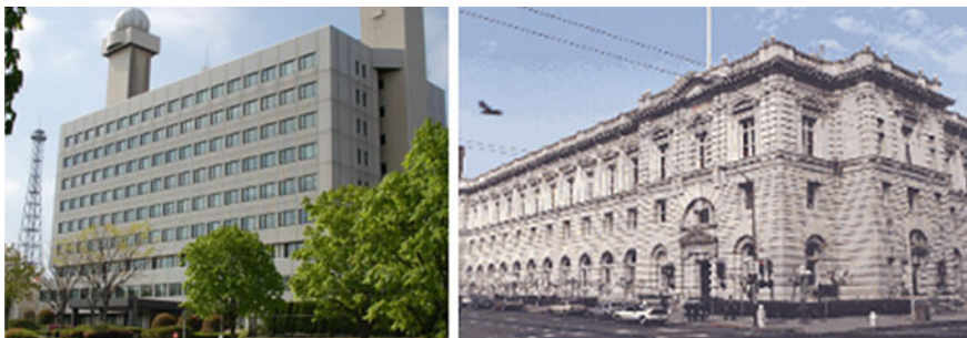
Fig. 24.9 Left: 9-story building in Sendai retrofitted with HDRB isolators. Right: 5-story US Court of Appeals building in San Francisco retrofitted with FPS isolators
