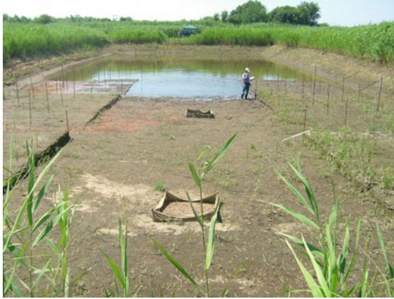
Fig. 20.14 A pilot experimental site to examine the effectiveness of topsoil removal by excavation on the recolonization of aquatic and short-lived wetland plants in the Watarase Retarding Basin. Photo by L. Hashimoto
