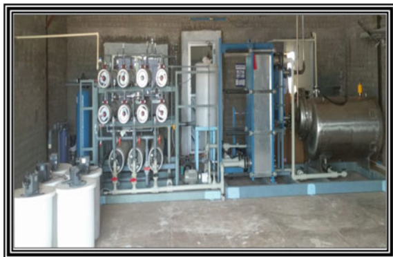
Fig. 9.3 Solar-biomass based multi-effect desalination (MED) system for coastal salinity in Narippaiyur, Ramanathapuram, Tamil Nadu
