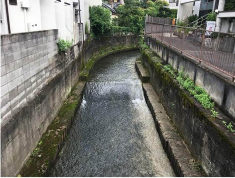
Photo 14.2 River as a function of water drainages. River was covered by concrete
