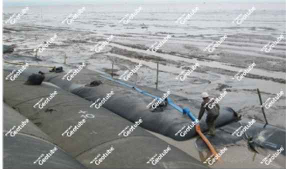
Fig. 11 Scour apron pumped to an inflated height of 0.5 m
