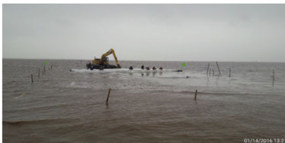
Fig. 14 High strength basal reinforcement over bamboo mattress
