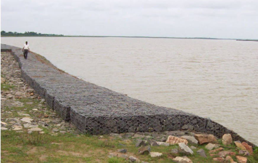
Fig. 19 Protection work on river Mahanadi
