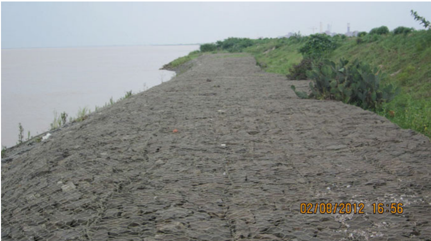
Fig. 20 Protection work on river Mahanadi after 10 years
