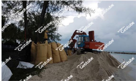
Fig. 25 Geobag lifting with spreader beam
