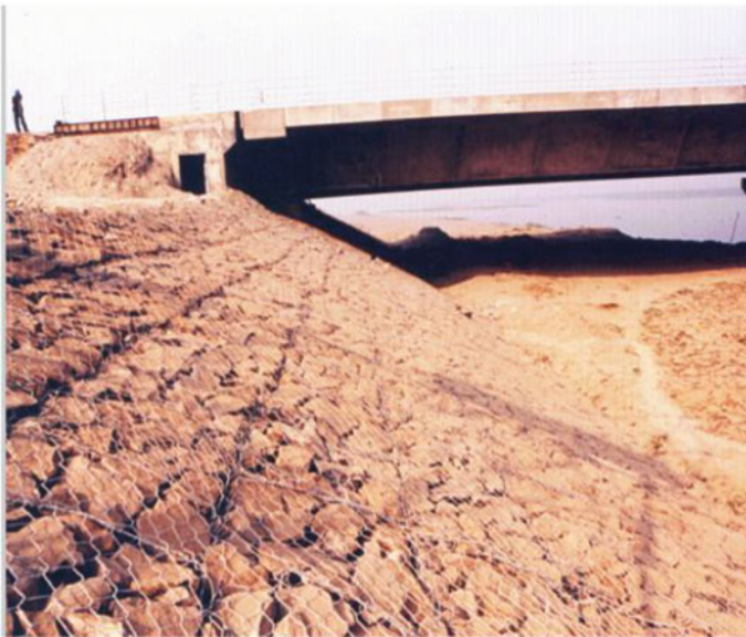
Fig. 21 Guide bund protection at Delhi Noida bridge 1999
