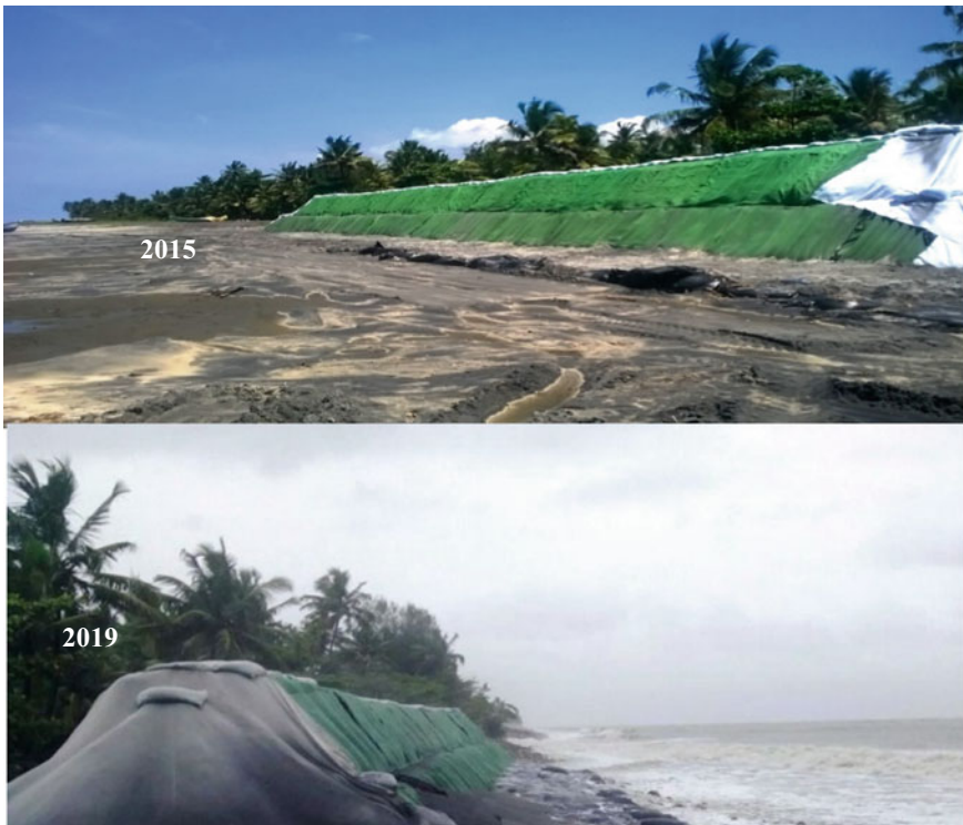
Fig. 11 A view of geo-synthetic seawall along Pallana, Kerala
