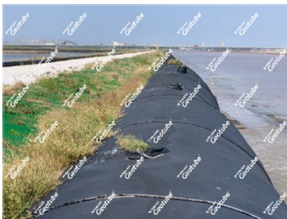
Fig. 16 Sand filled mattress covered with vegetation after 9 months
