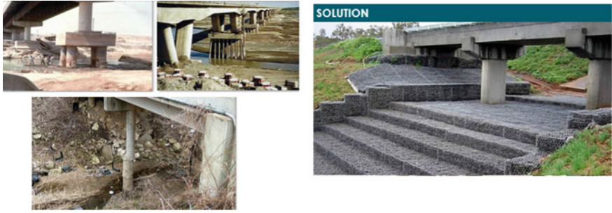
Fig. 7 Bridge abutment, pier, and floor protection
