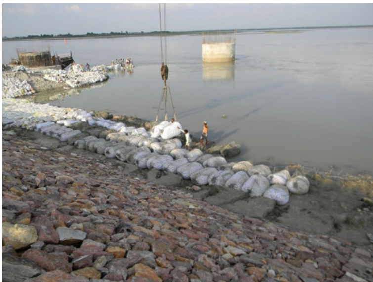
Fig. 23 Protection work with sack gabion filled with sand at Gopalganj
