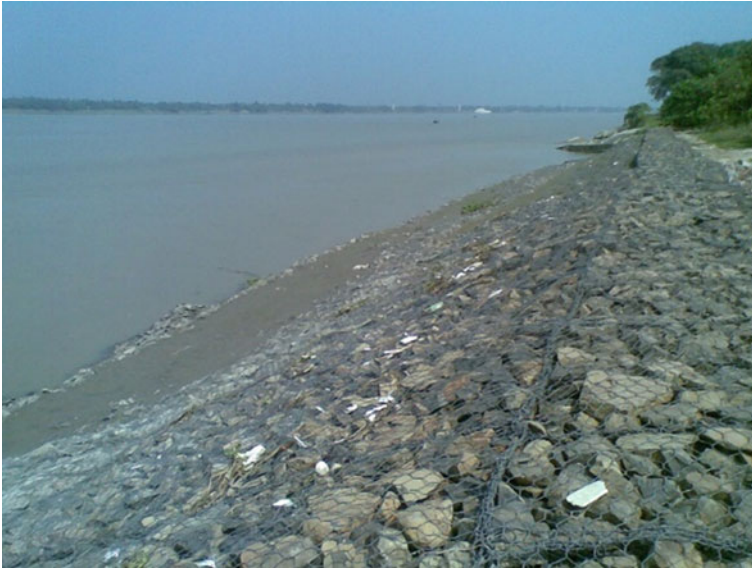
Fig. 24 Protection work with mattress at budge budge
