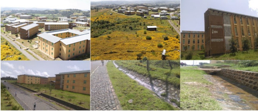
Fig. 2 Various buildings in study area with sloped roof and suitably connected to channels with pipes to conserve rainwater
