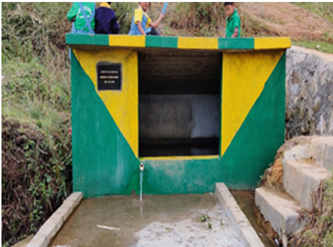
Fig. 2 Spring tap chamber is constructed to store flowing water from the Wahskur Sister spring, Village: Khelirihat, Meghalaya
