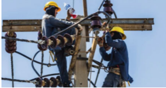
Fig. 1 Workers find faults in the transmission lines by climbing the transformer
