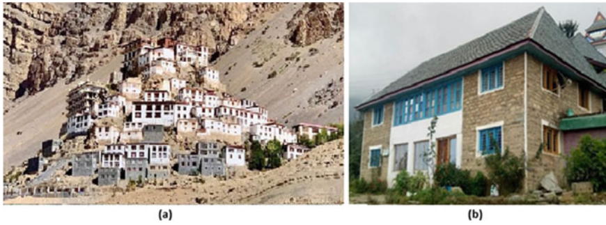
Fig. 1 a Kii monastery in village Kii in Lahaul and Spiti district of Himachal Pradesh. b Typical stone masonry house with sloping roof in Himachal Pradesh
