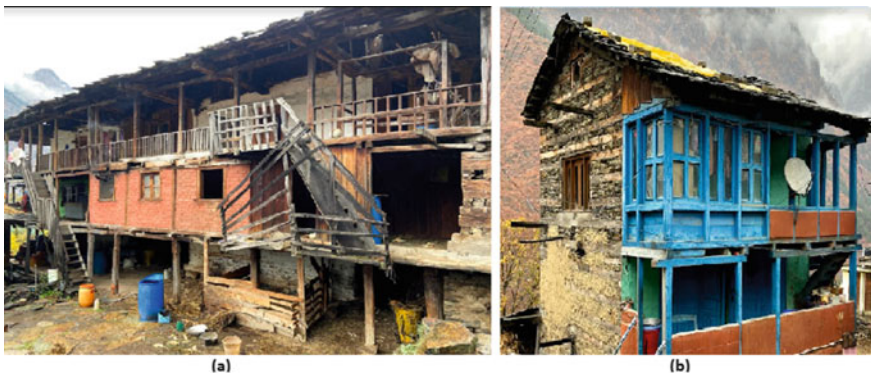
Fig. 8 Residential Kath-kuni structure
