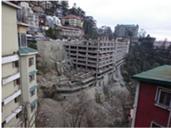
Fig. 4 Multilevel parking, lift
