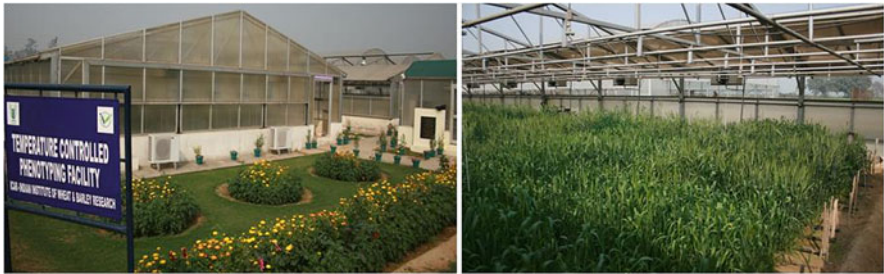
Fig. 20.2 Novel temperature-controlled phenotyping facility at ICAR-IIWBR, Karnal, Haryana, for precision phenotyping under temperature stress
