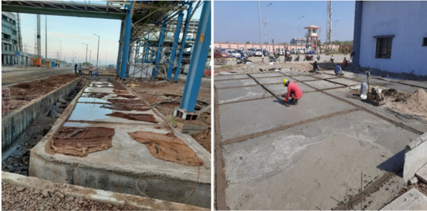
Fig. 11 Road segment cast at NTPC Khargone
