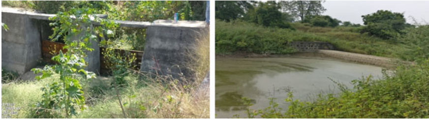
Fig. 2 Water harvesting structures in Junewani watershed
