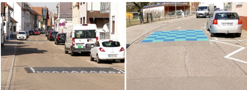
Fig. 10 Installation of humps and paintings in test tracks
