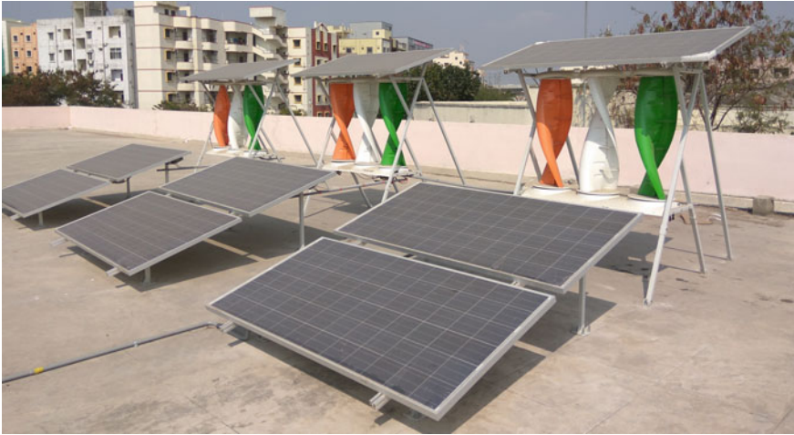
Fig. 11.3 Real-time installation of hybrid SPV and WECS
