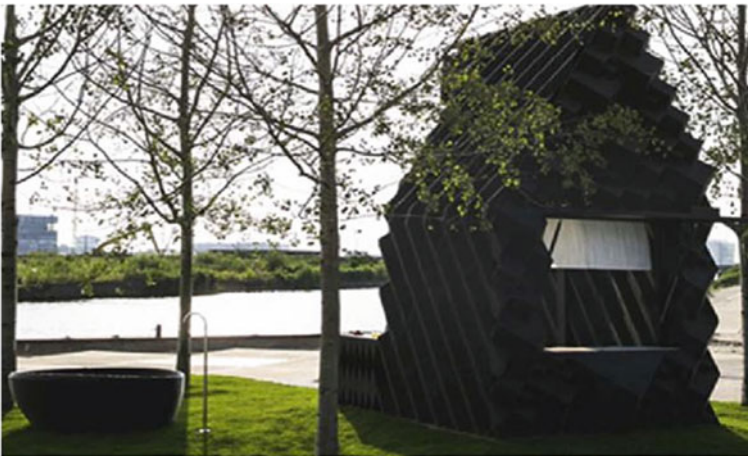
Fig. 4 First 3D-printed house by DusArchitects [17]
