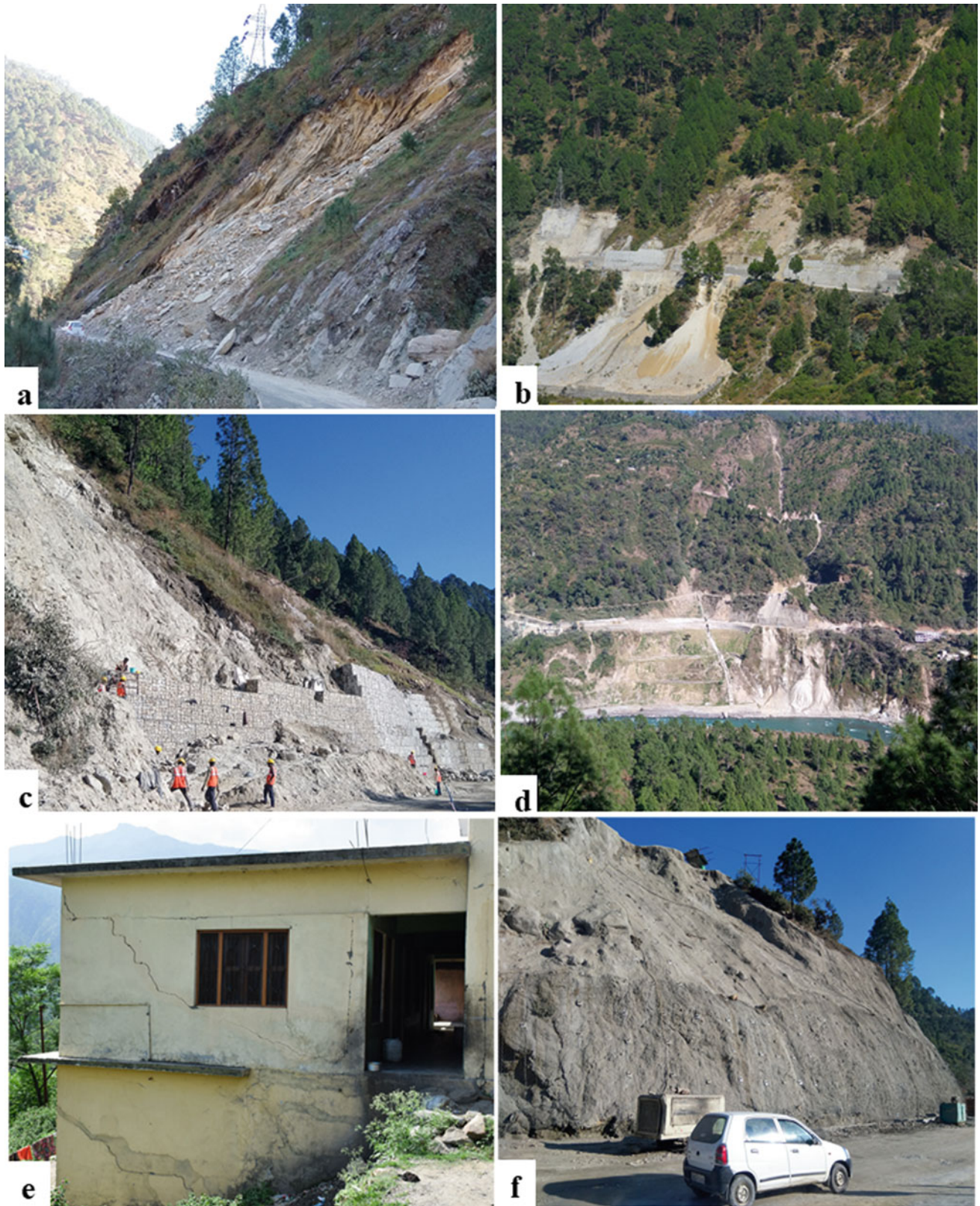
Fig. 4 a NH-7 damaged due to landslide (L1) present near Nandprayag town; b NH-7 damaged due to landslide (L2); c Rock bolting and gabion wall are preparing by NH workers for mitigation measure at landslide (L2); d Damaged house and road due to Landslide
