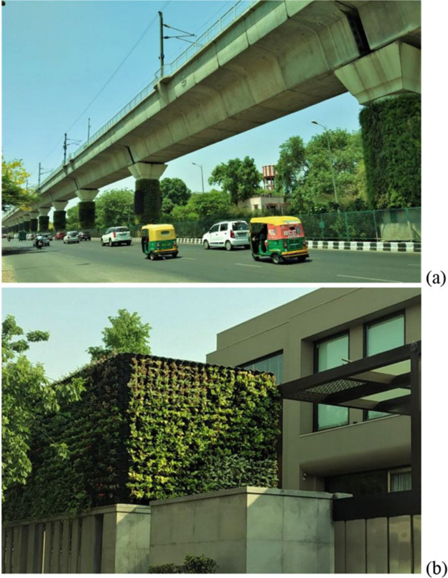
Fig. 3.3 Examples of urban greening in Delhi through non-food UA systems: (a) vertical gardens constructed on Metro rail pillars by the state government, and (b) green wall in a privately owned residential household. (Source: author)
