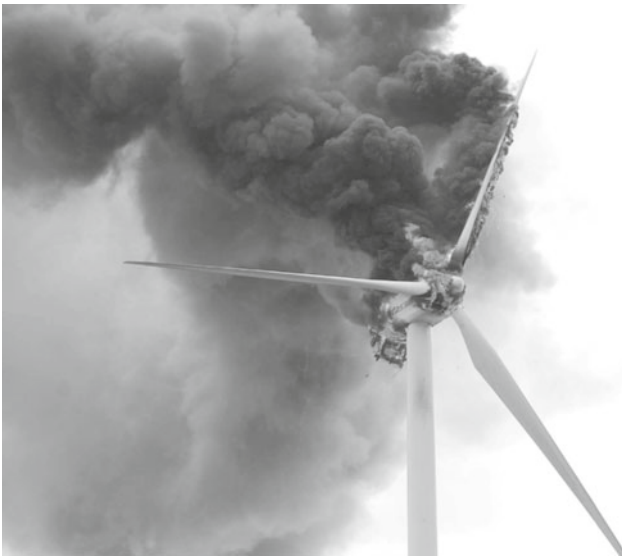
Fig. 20 Burning wind turbine as result of a lightning strike [21] (NDR)
