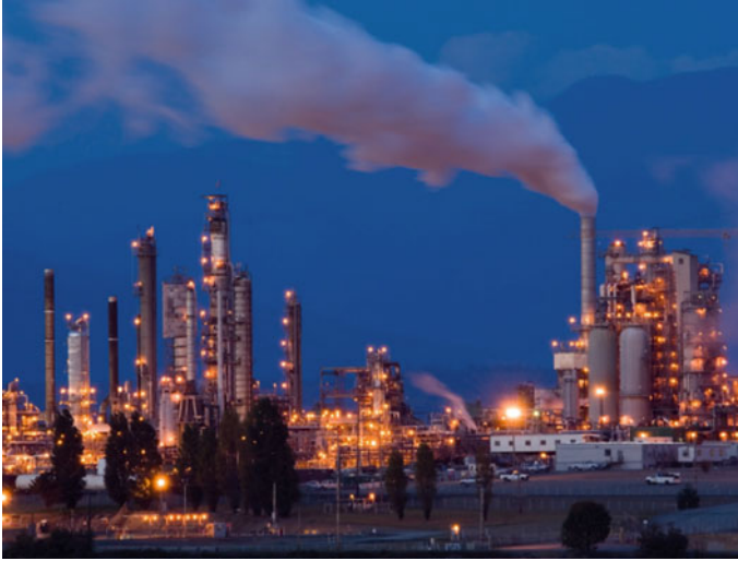
Fig. 4 Petrochemical plant inherently selfprotecting for tall structures. Non-isolated protection are normally applied in order to divert the striking point from metal structure to be protected. Adapted from Tompson [6]
