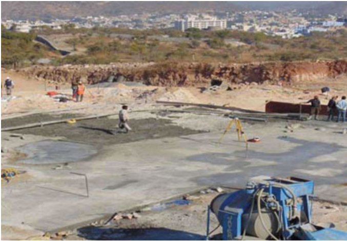
Fig. 8 Foundation level preparation
