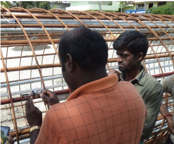
Fig. 1 Strain gage installation in progress
