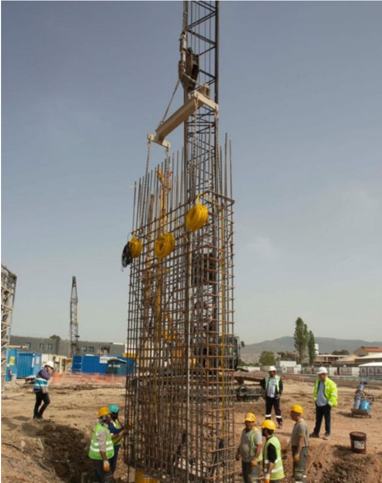
Fig. 1 Barrette installation
