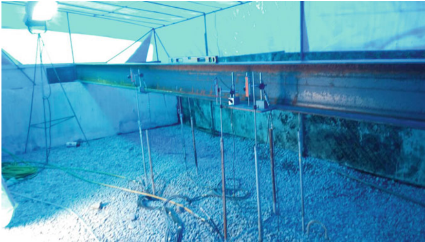
Fig. 2 Barrette load test set up
