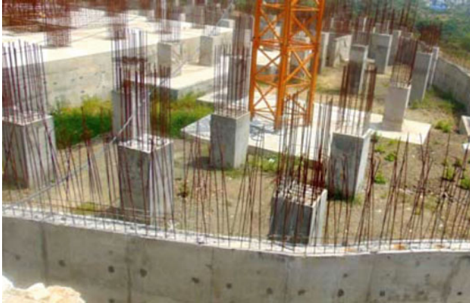
Fig. 9 Foundation construction in progress
