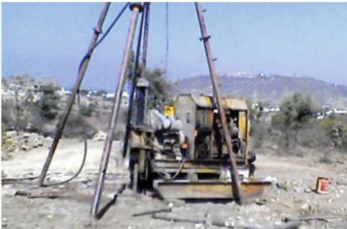
Fig. 5 Drilling in progress
