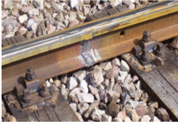
Fig. 1 An alumino-thermit weld on rail
