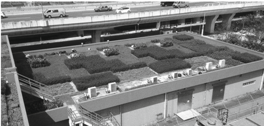
Fig. 11.21 Green roof at Shatin Sewage Treatment Works (Modified from: DSD)
