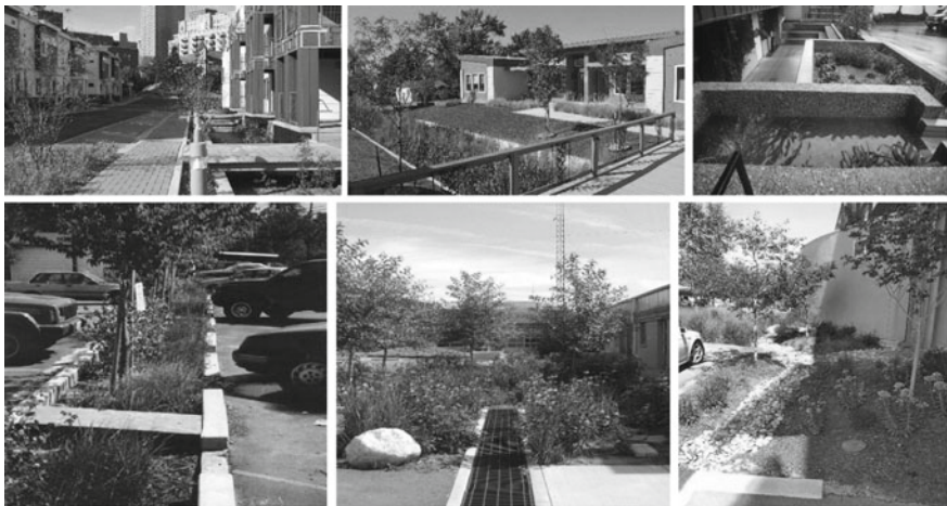
Fig. 11.23 Rain gardens, porous pavements, and planter box techniques in Denver, CO, USA, for stormwater management (Modified from: Agency 2017)
