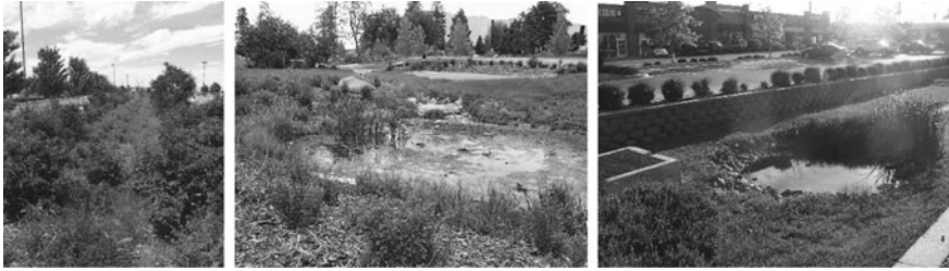
Fig. 11.24 Bioswale and detention/retention pond techniques in Denver, CO, USA, for stormwater management (Modified from: Agency 2017)
