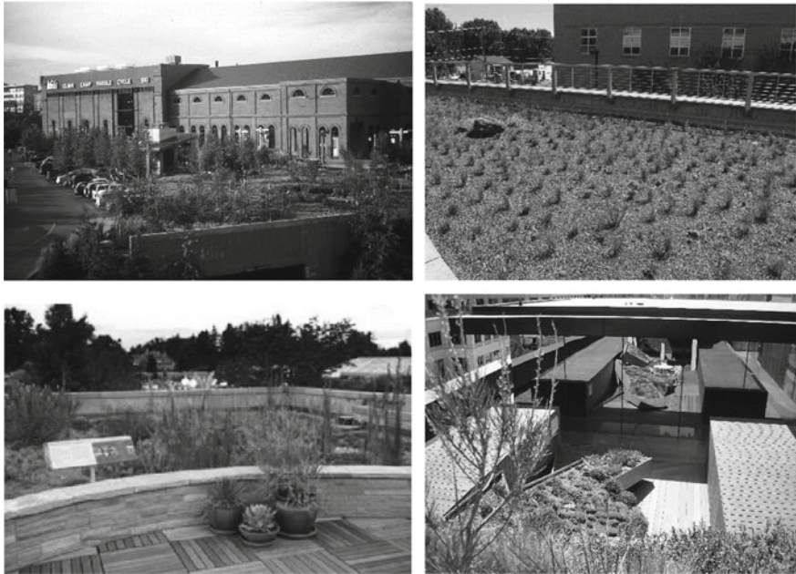
Fig. 11.22 Green roof technique in Denver, CO, USA, for stormwater management (Modified from: Agency 2017)
