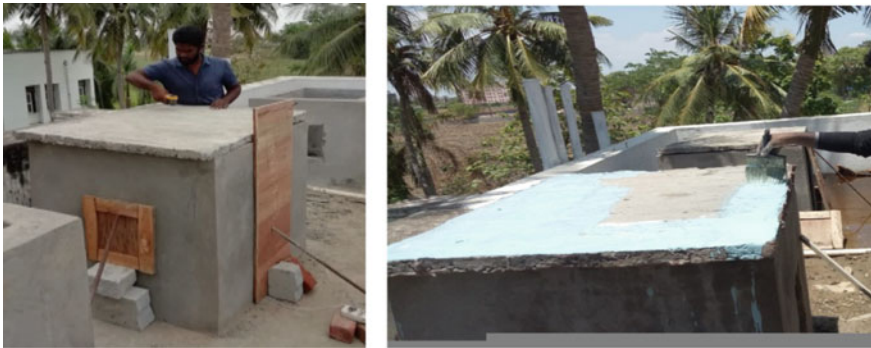
Fig. 4 Application of acrylic cool roof coating over the roof portion
