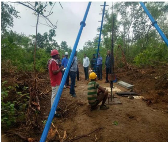
Fig. 1 SPT test on the proposed original foundation site
