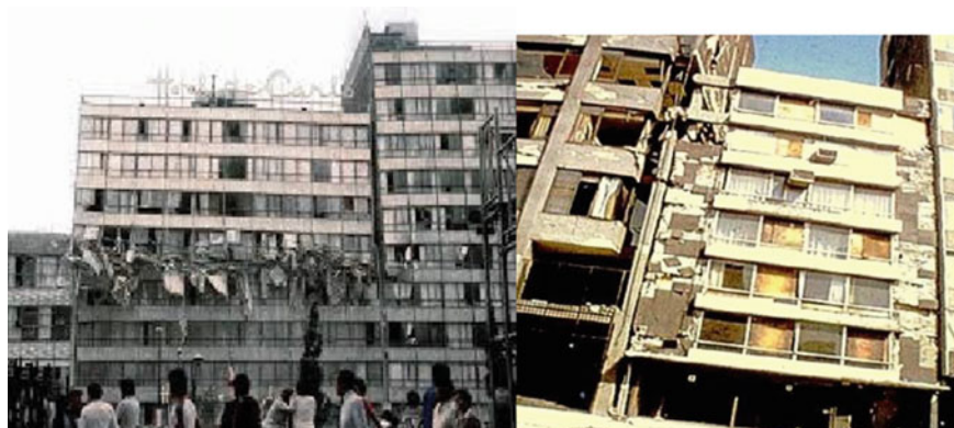
Fig. 2 Pounding damage during Mexico earthquake 1985. Source http://www.smate.wvu.edu/teched/geology/eq-Mexico.html
