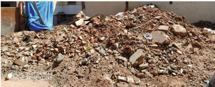
Fig. 2 Construction and demolition waste disposed in an abandoned site
