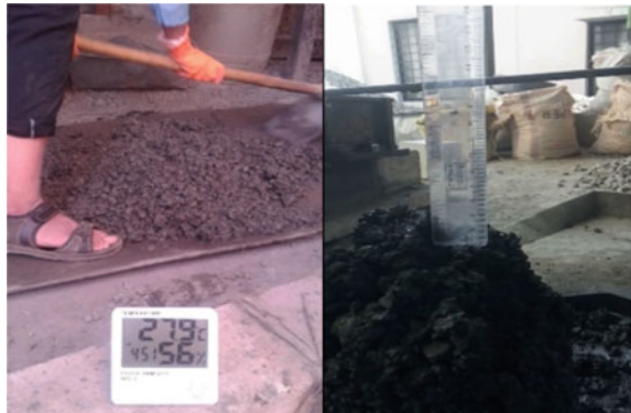
Fig. 2 Concrete mixing with slump test to control on workability
