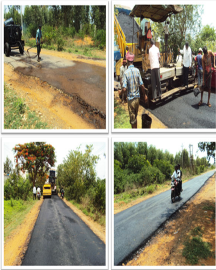
Fig. 6 Various stages of test track overlay
