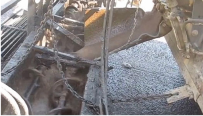
Fig. 1 Material discharge plate of microsurfacing machine
