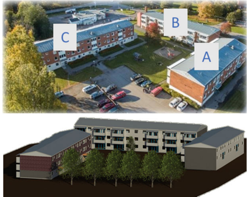
Fig. 14.1 Three buildings in the cluster for renovation in Ludivika, Sweden
