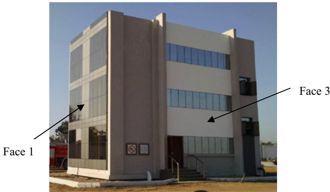
Fig. 7 Full-scale façade fire experimental facility at IIT Gandhinagar [27]
