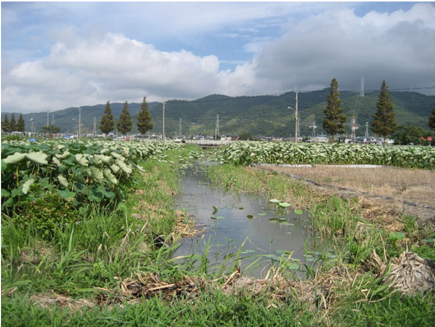
Fig. 4.7 Before renovation work of an enta -type dikes
