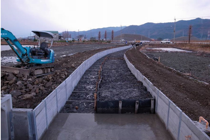
Fig. 4.8 During renovation work of an enta -type dikes
