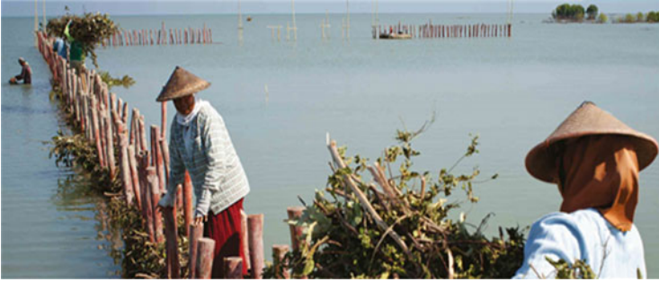
Fig. 17.2 ‘Building with Nature’ activity at Timbul Sloko village, Indonesia (Source: Spalding et al. 2014b)
