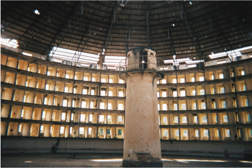
Fig. 7 Inside one of the prison buildings at Presidio Modelo, Isla de la Juventud, Cuba. I, Friman [GFDL ( http://www.gnu.org/copyleft/fdl.html ), CC-BY-SA-3.0 ( http://creativecommons.org/licenses/by-sa/3.0/ )]
