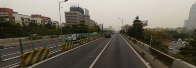
Fig. 3 Jiangwan Interchange (elevated road)
