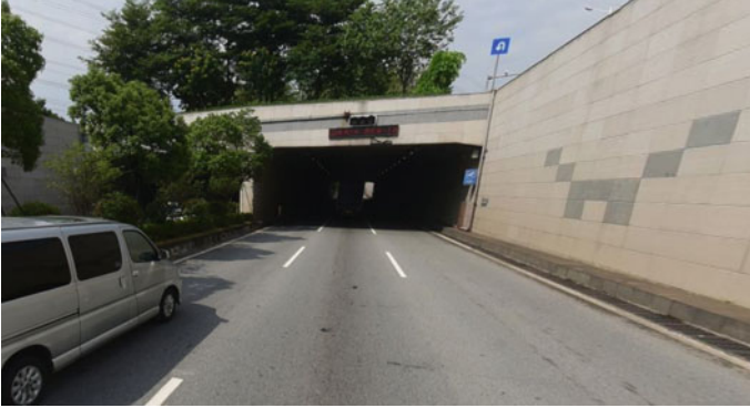
Fig. 1 Huakou Tunnel (underpass tunnel)
