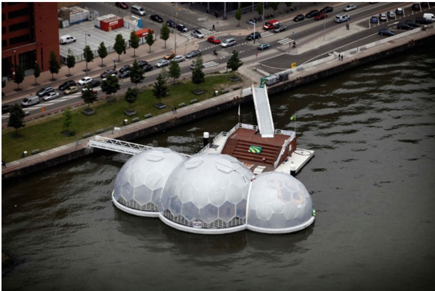
Fig. 2 Rotterdam Floating Pavilion, The Netherlands
