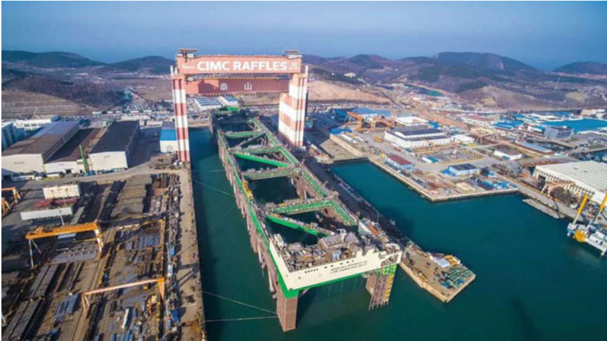
Fig. 12 Havfarm 1 launched at yard in China
