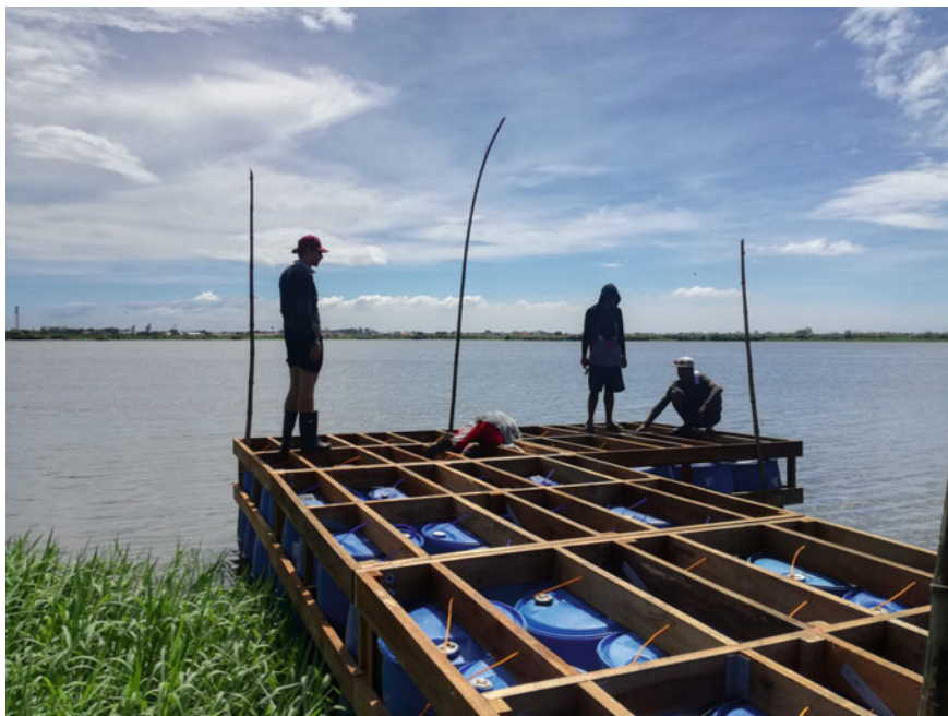
Fig. 6 Floating foundation modules
