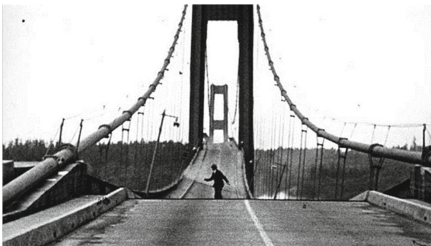
Fig. 1 Tacoma bridge excessive vibrations. Source https://www.thestructuralengineer.info/education/bridge-management/bridges/tacoma-narrow-bridge-collapse
