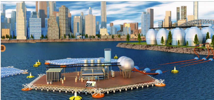
Fig. 8 Floating solar powered desalination plant on Sea6’s Dweep tensegrity based platforms [25]
