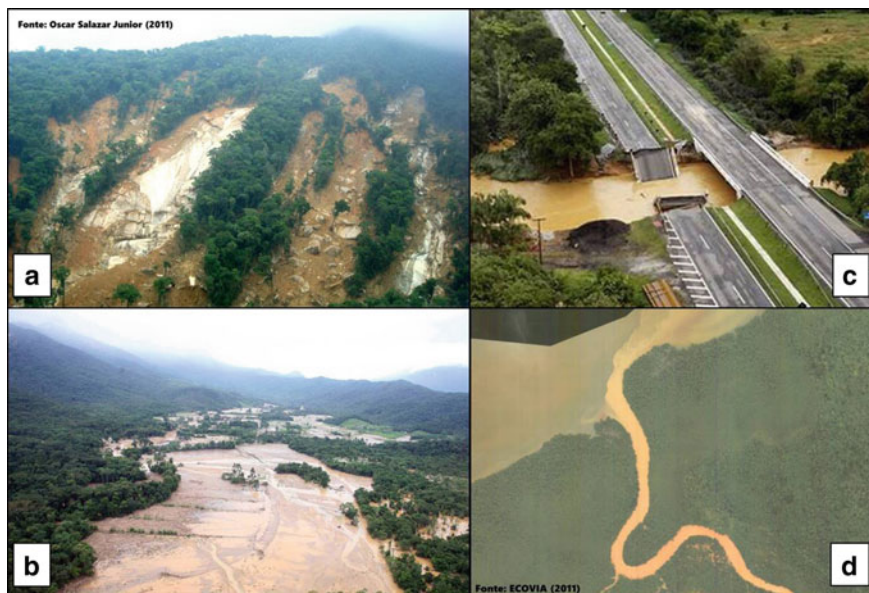
Fig. 8 Results of the extreme rainfall event of 11/03/2011. a Translational landslide in the mountains. b Floods and burials at the alluvial plain of the Jacareí River. c Breaking of the bridge at the BR 277 highway, draining a part of the material at Antonina Bay. d Discharge of the material at Antonina Bay. Source a—Oscar Salazar Junior, 2011; b—Rogério Machado/SECJ, 2011; c—Orlando Kissner/Agência Estadual de Notícias, 2011; Estate News Agency, 2011 and d—Ecovia, 2011)
