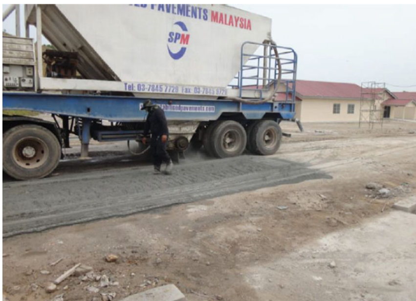
Fig. 2 Spreading of the cement using mechanical spreader
