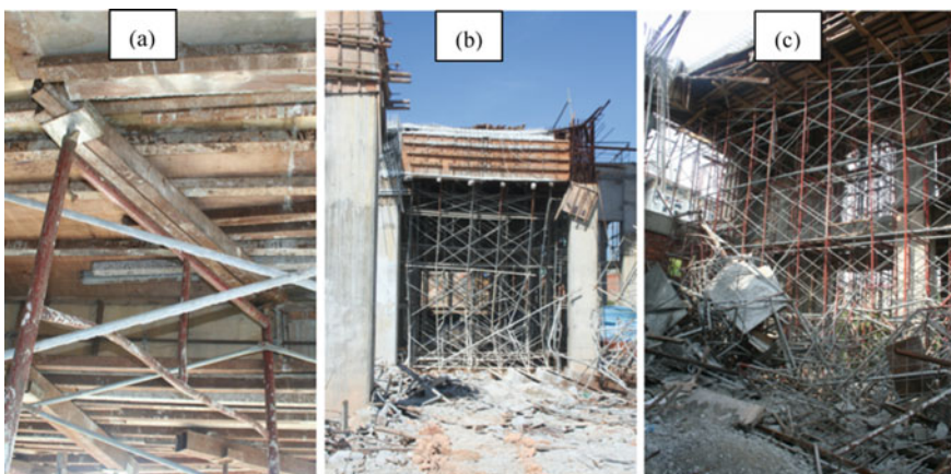
Fig. 5 Frame scaffold erection a Case 1 [15] b Case 2 [7] c Case 3 [1]
