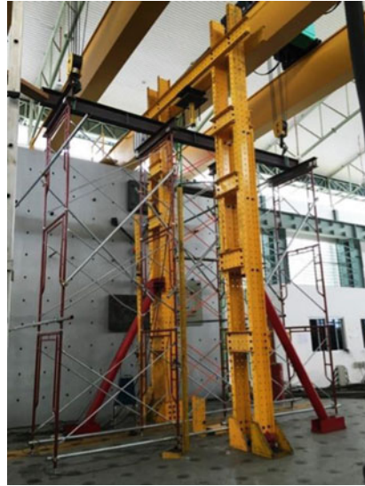
Fig. 7 Frame scaffold erection on test equipment
