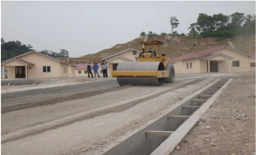
Fig. 5 Compaction using steel drum roller
