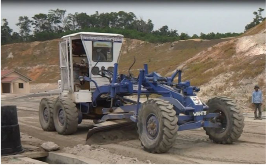
Fig. 4 Trimming of the surface using grader
