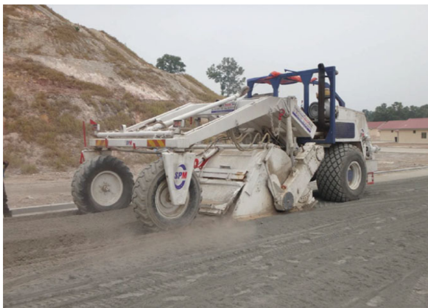
Fig. 3 Dry mixing process using stabiliser machine
