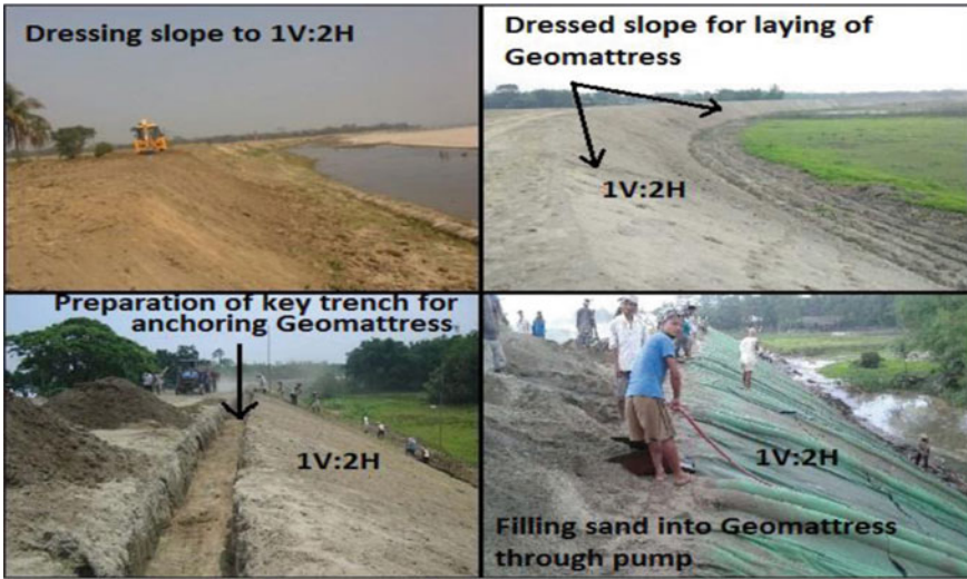
Fig. 7 Installation of Geotextile mattress at various stages
