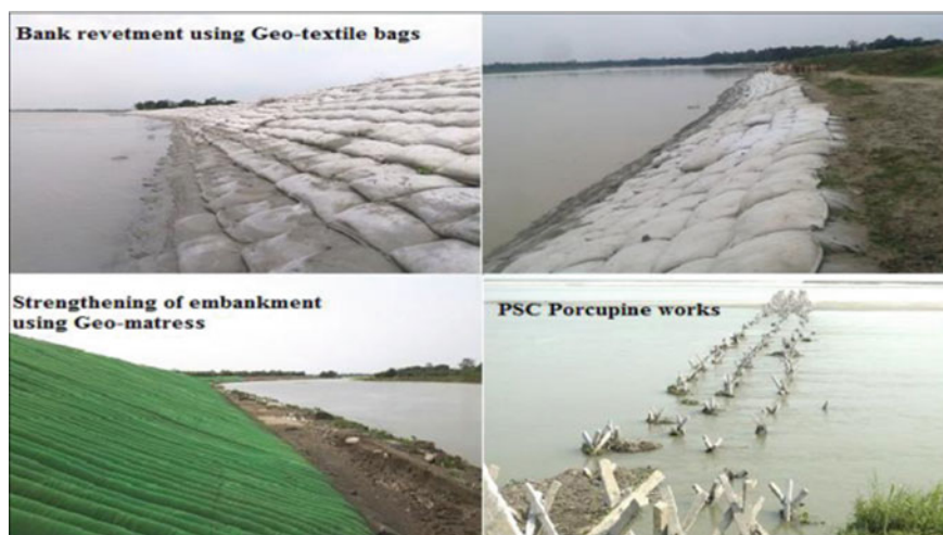
Fig. 4 Implementation of Geotextile bags, Geo-matress and PSC Porcupine works
