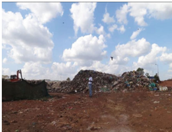
Fig. 2 Waste landfill site at Turamuri
