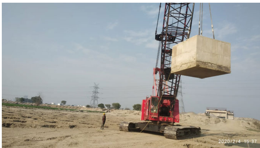
Fig. 6 Dynamic compaction at the site in progress
