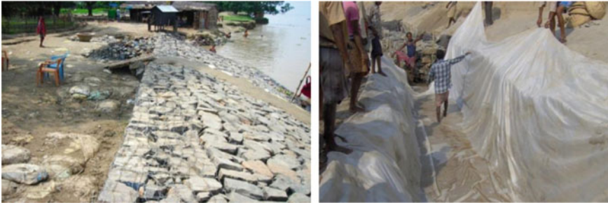
Fig. 11 Anti-erosion works at Farakka Barrage Project, West Bengal
