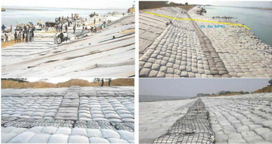
Fig. 2 Placement of the filter media, Geobags and Polypropylene Rope Gabions
