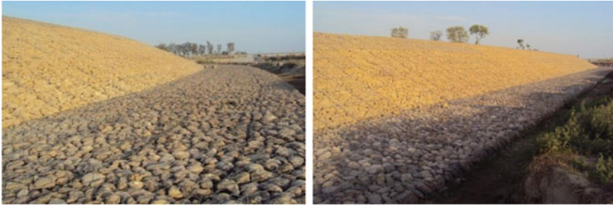
Fig. 6 Completed embankment in Phase II
