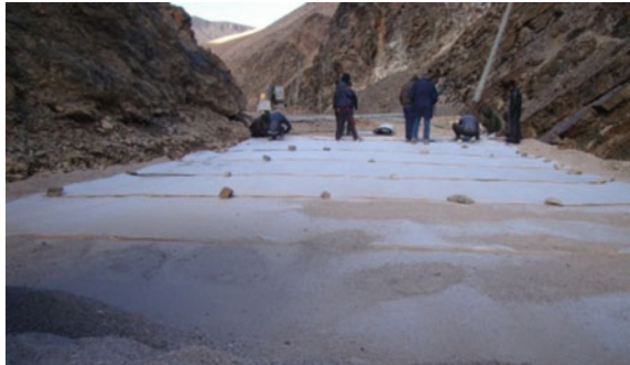
Fig. 7 GCD laid in slope and being covered by sand layer
