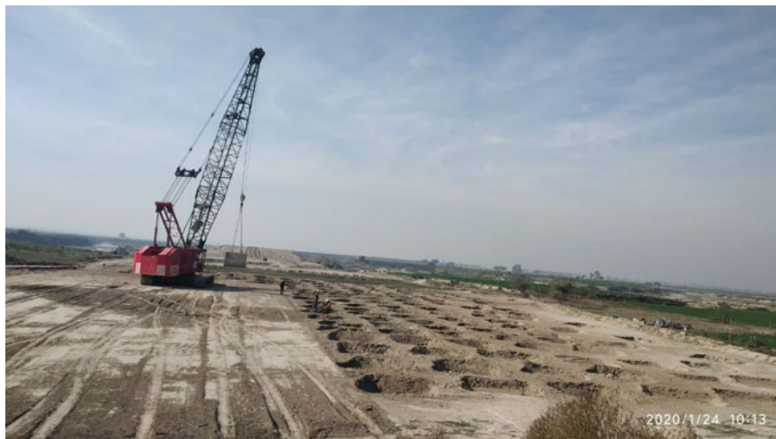
Fig. 5 Dynamic compaction at the site in progress
