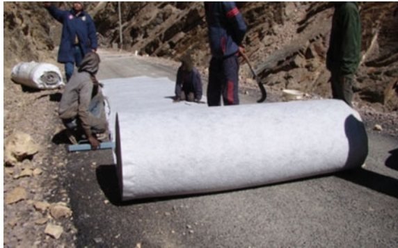
Fig. 6 Geocomposite drain being rolled out for cutting
